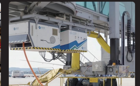
Hangzhou International Airport
