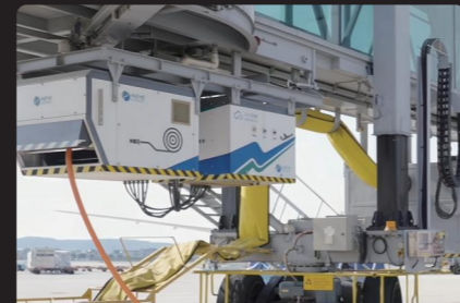
Hangzhou International Airport
