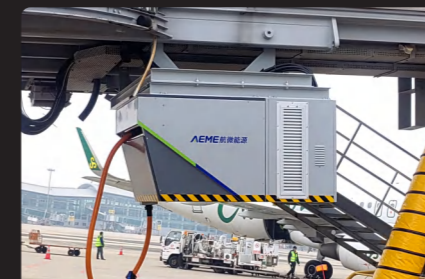
Nanchang International Airport
