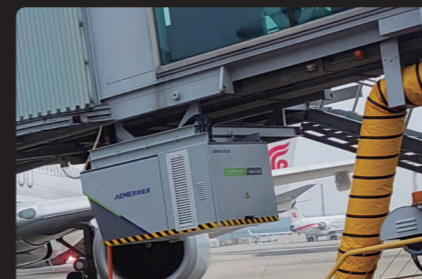
Nanchang International Airport
