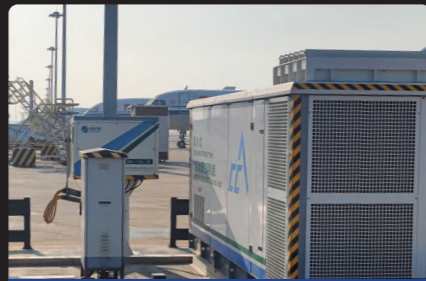
Shijiazhuang International Airport
